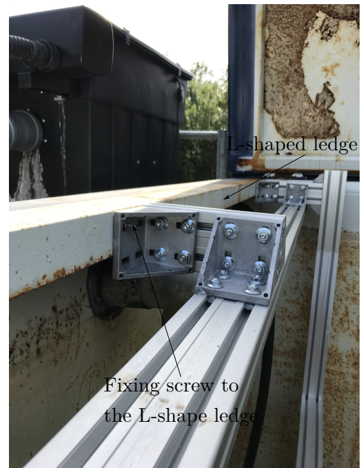
(b) Image of the framework screwed on the L-shaped ledge
